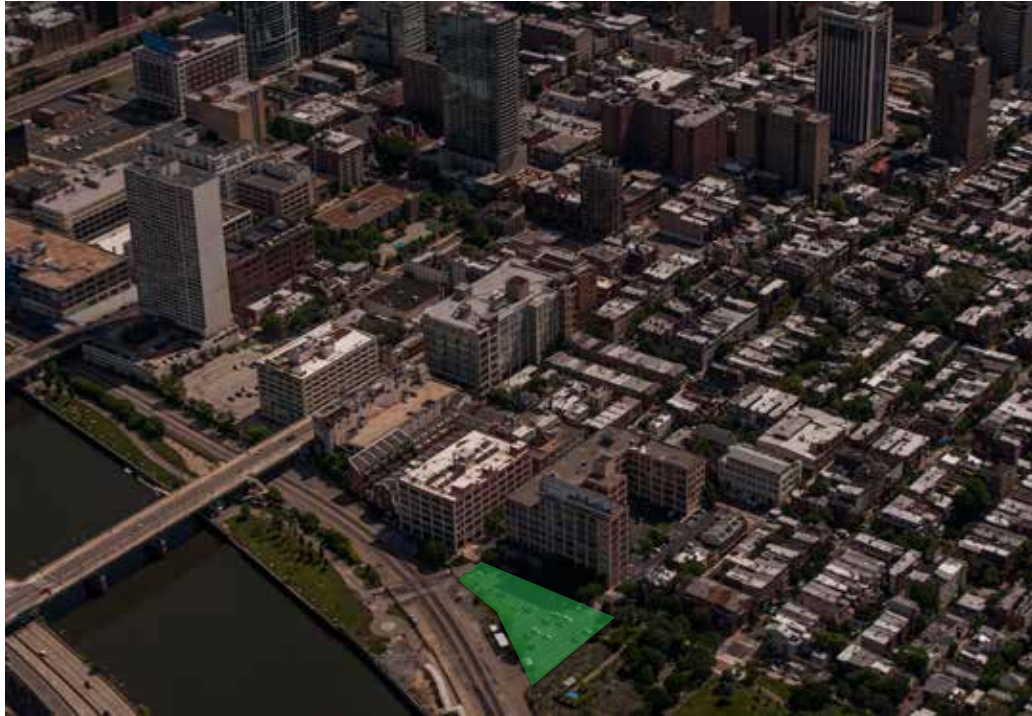
Aerial View from Southwest
